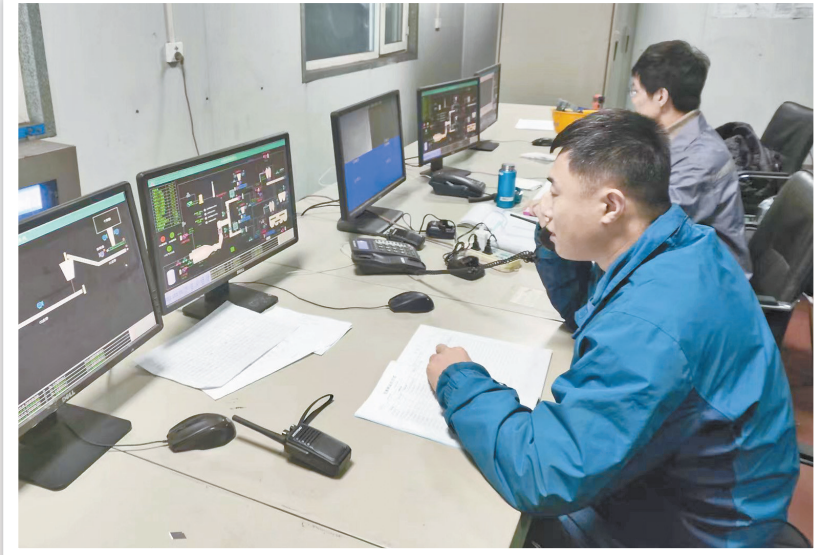
▲城西热源厂制粉车间监盘
